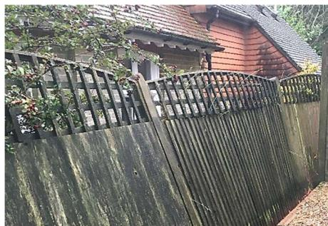
The fence between the church and our neighbour (Old Vicarage West) has been blown off vertical during the recent storm. It has been arranged for a fencing contractor to inspect the damage before deciding on a solution. A second quotation will be obtained.
